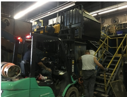
Image 3. Installation of new Eddy Current
