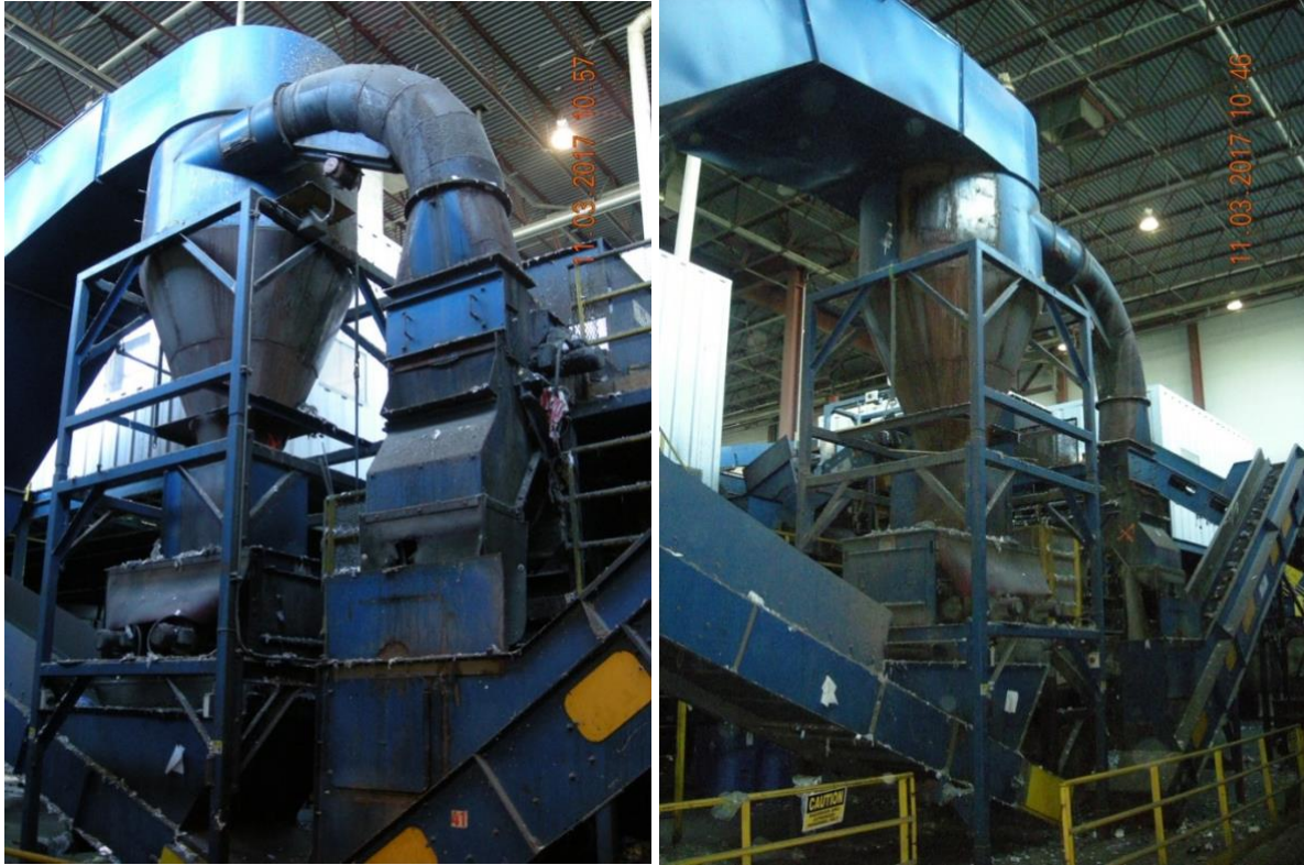
Figure 4: Air Separator Cyclone and Glass Screen Before Removal
