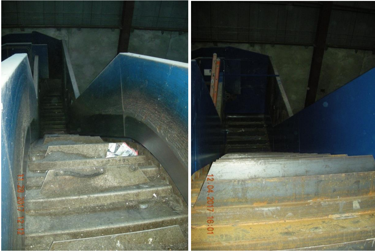
Figure 3: In-Feed Conveyor Pre and Post Upgrade
