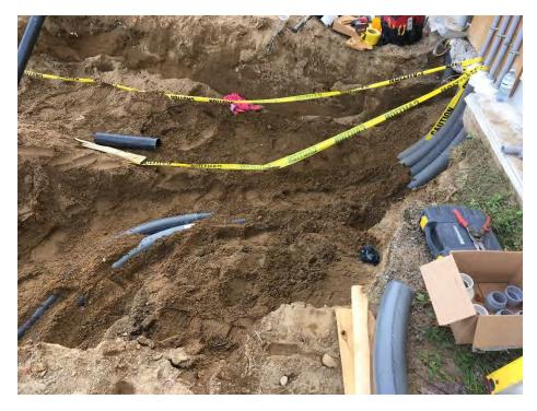
Photo 10 (Sep21-16) Installation of electrical requirements for Blue Box recycling stationary compactors.
