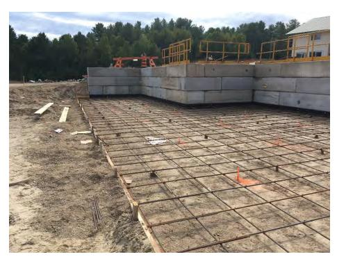
Photo 13 (Sep29-16) Rebar installation in advance of installation of new concrete pad.
