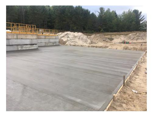
Photo 14 (Sep30-16) New concrete pad for Blue Box recycling stationary compactors.
