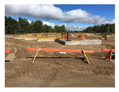
Photo 12 (Sep23-16) Final backfilling of new granulars for reconstructed retaining wall.
