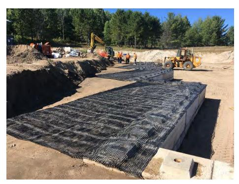
Photo 11 (Sep20-16) Geogrid installation for new retaining wall.
