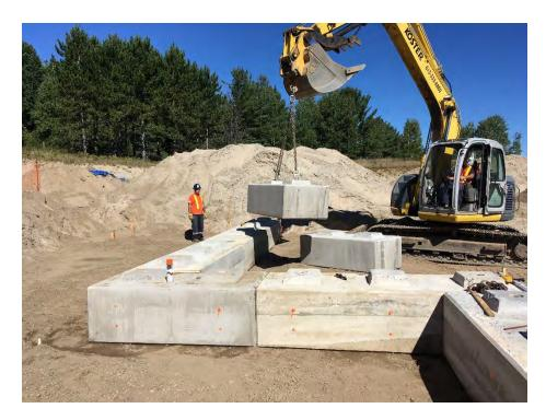
Photo 8 (Sep15-16) Progressive emplacement of new retaining wall blocks.
