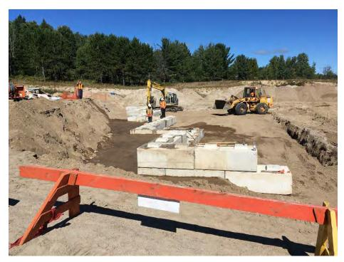
Photo 7 (Sep15-16) New retaining wall construction and progressive backfilling.
