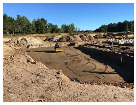
Photo 6 (Sep12-16) Installation of new granulars in advance of new retaining wall and concrete pad contruction.
