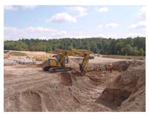
**Photo 5** (Sep07-16) Project start including sub-excavation in advance of new granular emplacement for new retaining wall.
