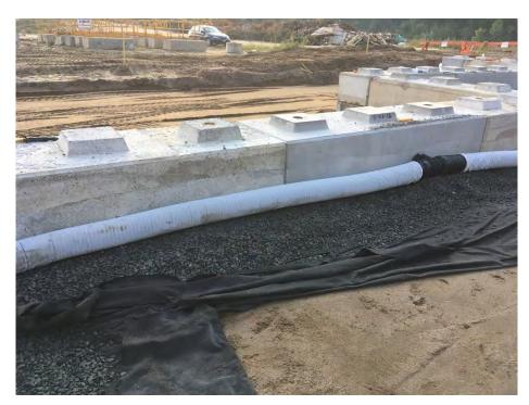
Photo 9 (Sep20-16) Installation of drainage enhancements for retaining wall.
