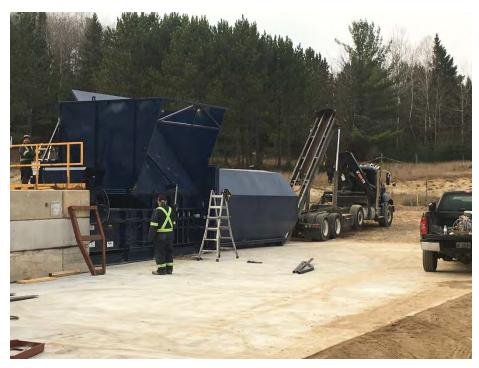
Photo 15 (Nov08-16) Delivery and installation of three (3) Blue Box recycling stationary compactors.
