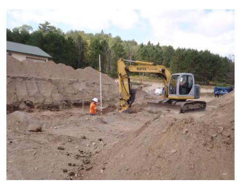
**Photo 4** (Sep07-16) Project start including sub-excavation in advance of new granular emplacement for new retaining wall.
