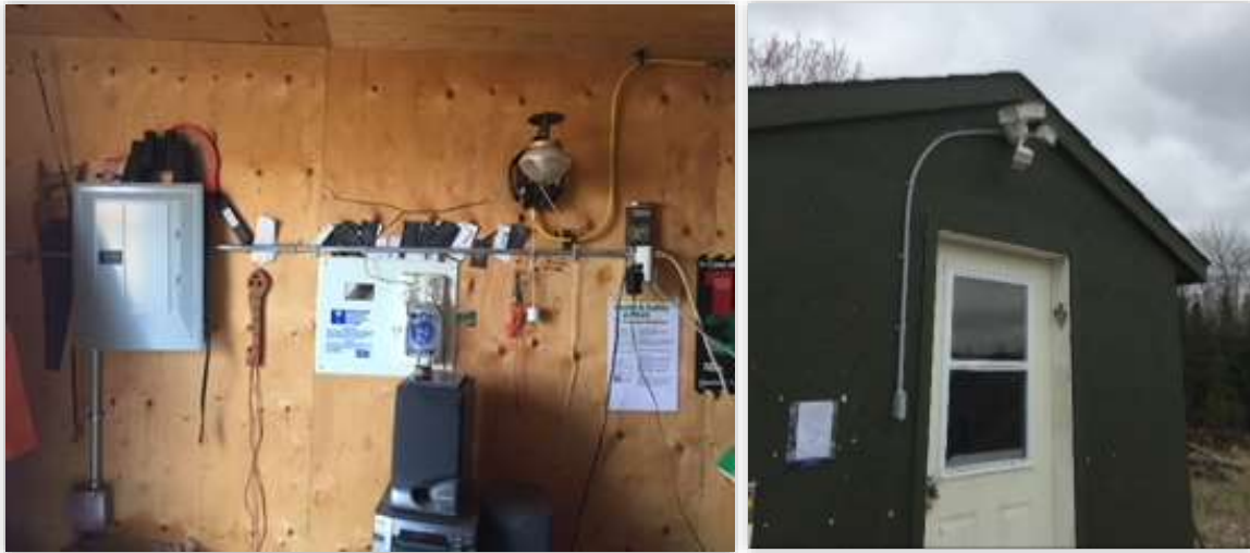
Figure 3: Spotter shack electrical improvements
