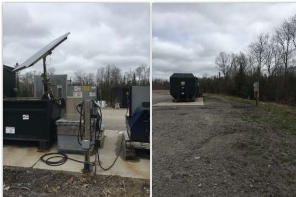
Figure 1: Photograph of electrical site upgrades
