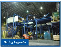
operating near capacity, combined with the need to add new materials to its blue box program and the planned implementation of a bi-weekly cart-based collection system in 2016, the Region completed a material recovery facility capital upgrade in 2014, at a cost of \$3.1 million. The upgrade resulted in annual savings of \$612,600; annual avoided costs of \$2.15 million and extended the facility's operating life to 2020
