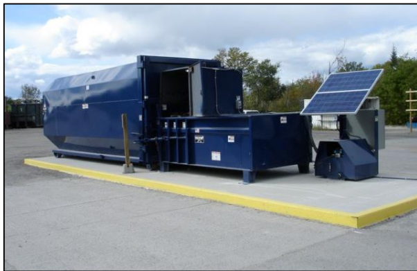
Figure 4: Concrete Pad Trip Hazard and Corrections
