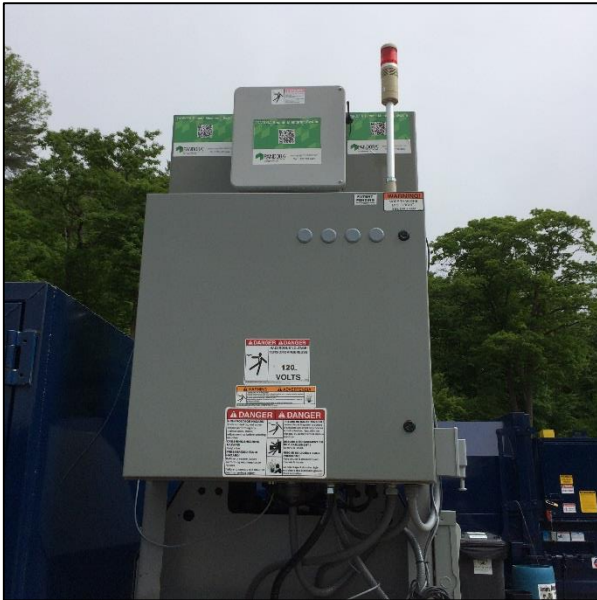
Top left: Video camera inside a material receiving enclosure, which allows attendant to monitor contents of enclosure prior to running compaction cycle. Top right: Example of video footage from within the enclosure. Bottom left: Pandora remote communications modem and electrical panel on compaction container.
