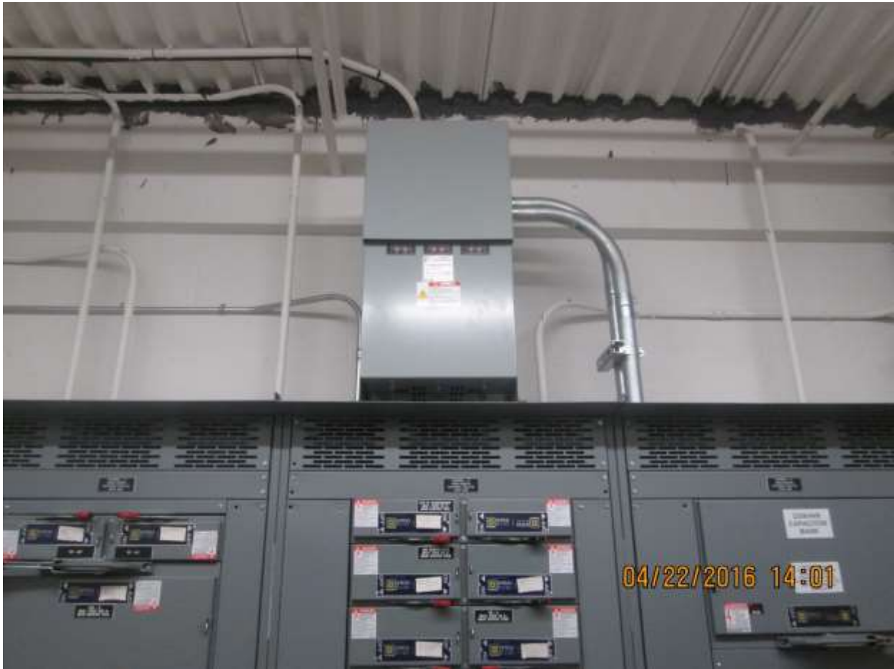
Figure 1: Installed Capacitor
