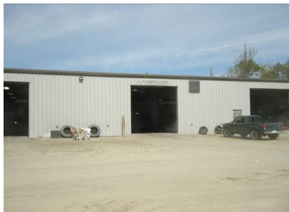
Photo 4 Exterior of MRF
