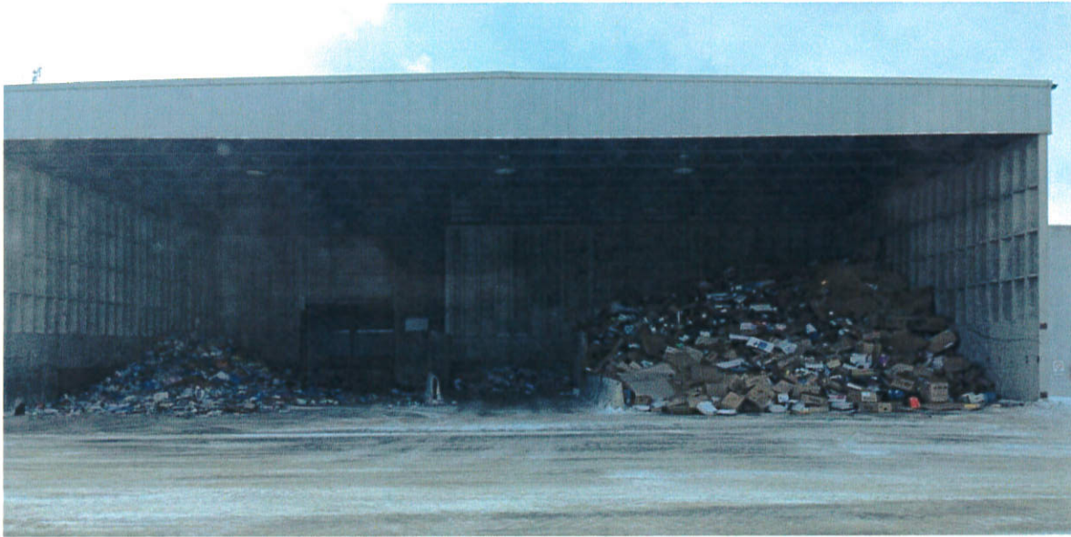
Recycle building for comingle, paper and cardboard at the Kenora Transfer Station
