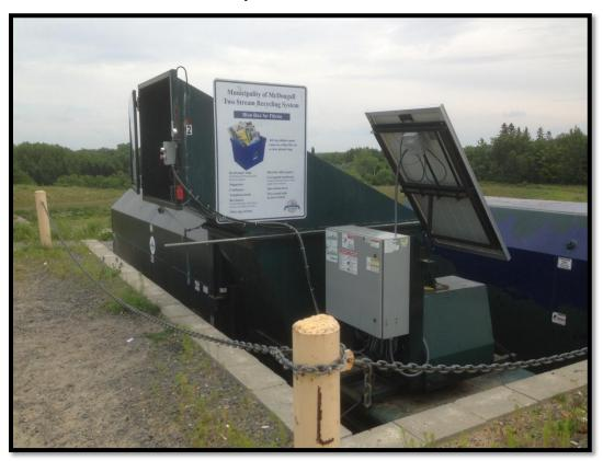
**Photo 2 Solar Powered Compactor**
