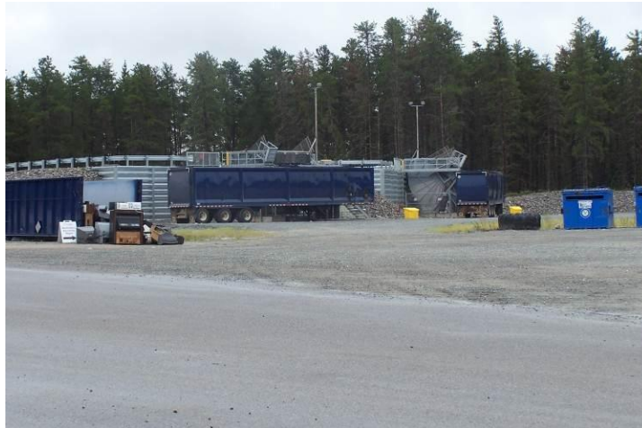
Photo 4 Transfer System at Deloro Landfill Site
