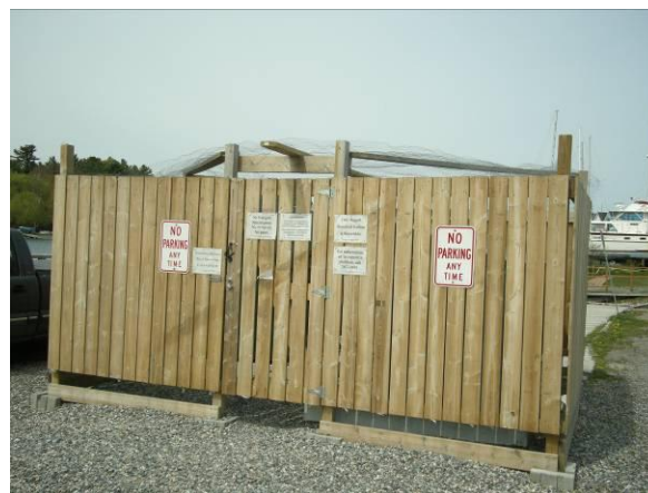
Photo 2 Public Drop off (Channel Street)
