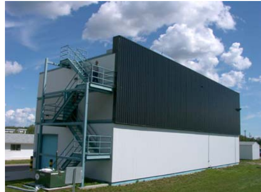
Figure 5.1: Solarwall, CFB Cold Lake, AB
