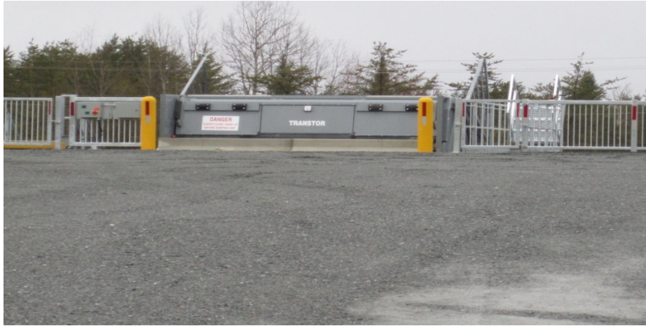
Figure 1: Transtor in place at Deloro Landfill
