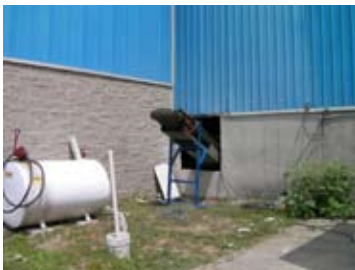
Placement of garbage conveyor June 19, 2009
