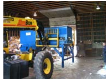
Placing Eddy Current into plant June 19, 2009
