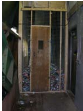
New UBC Bunker June 10, 2009
