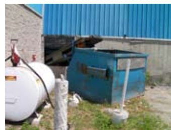
Garbage conveyor and bin June 22, 2009
