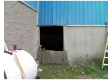
Cutting hole for garbage conveyor June 19, 2009
