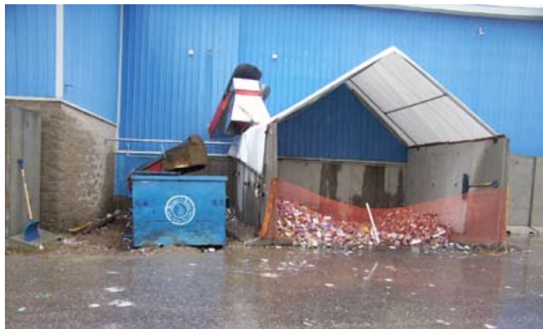
Above shows the bunker built to keep rain and snow off steel.
